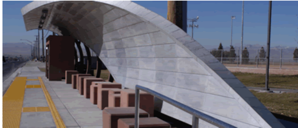
Figure 4.9 Typical MAX Station
